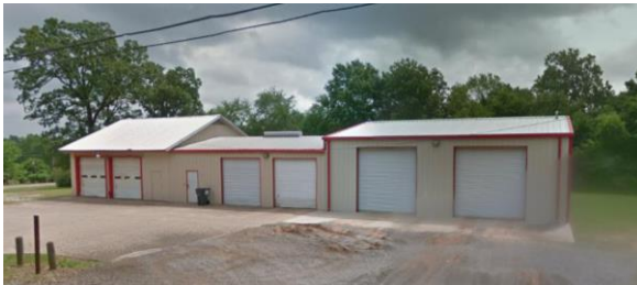
Figure 127: Jackson Heights VFD, Station 1
